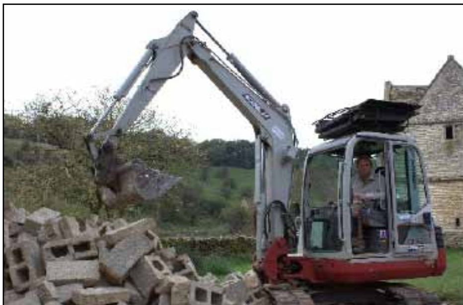
Josh Harrison of Four Shires Construction during the removal of the Tractor Shed in October 2009
