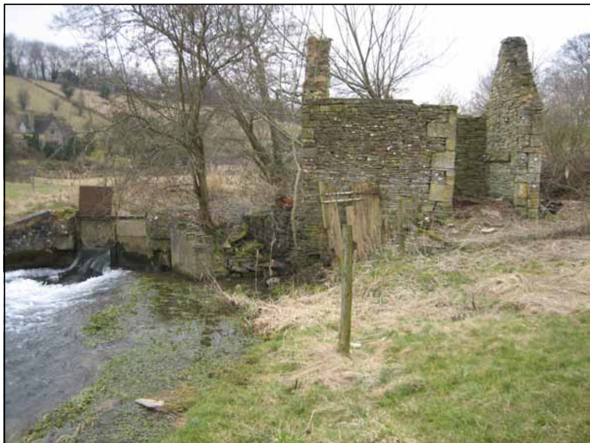
fig 5 – Turbine shed, sluice gate and exit channel for leat – current condition
