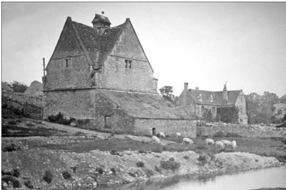
fig. 1 Lean-to in early 1900s showing window for access for maintenance of wheel on south elevation and 45° Welsh slate pitch roof
