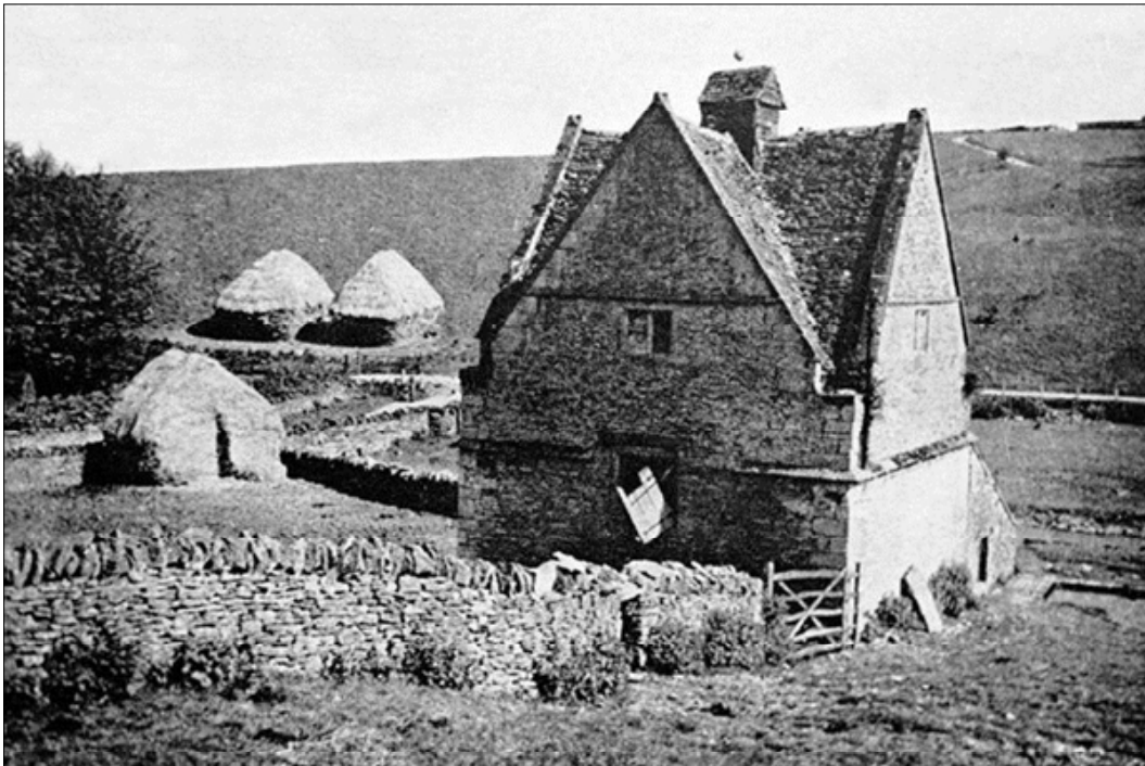
fig. 3 North elevation - showing the wooden door which was inserted to give access to the first floor storage area for grain
