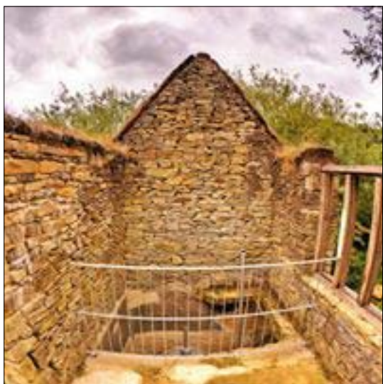
The turbine shed after restoration (Dovecote Day 2018)
