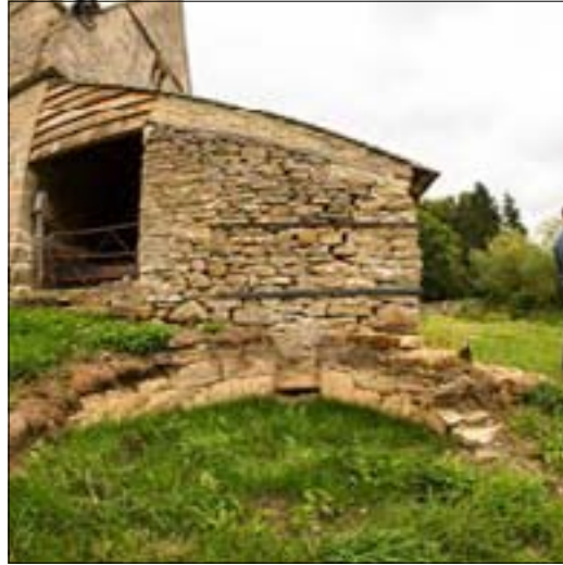
Horseshoe headrace to lean-to (Dovecote Day 2018)
